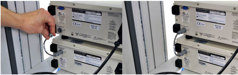
Figure 9: Installation of Footswitch Jumper cable between the ASU and ASB.
